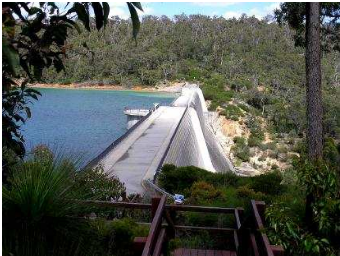
New Victoria Dam (opened Nov. 1991)
