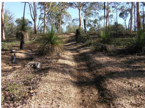
Gravel displaced widely around track (within Wandoo Nat. Park)
